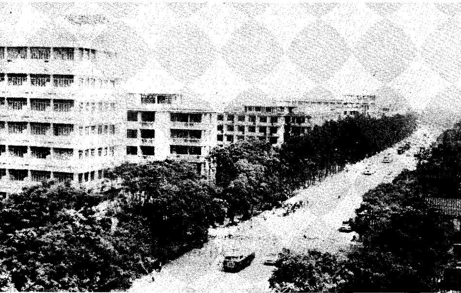
May Day Boulevard after being widened.
